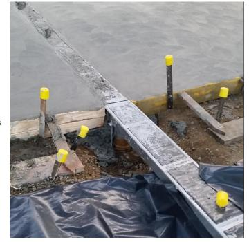
covering the drain bowl with a suitable covering, PVC (also known as grey) tapes, builders plastic wrap, foams and plywood materials all of which are suitable to be used with stainless steel for the duration of the construction.
